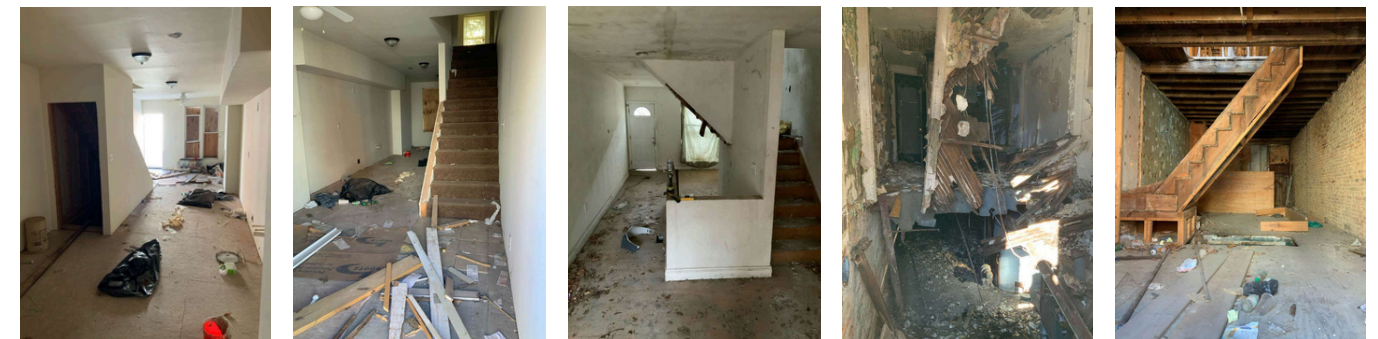
Exterior Views of Misc. Units
